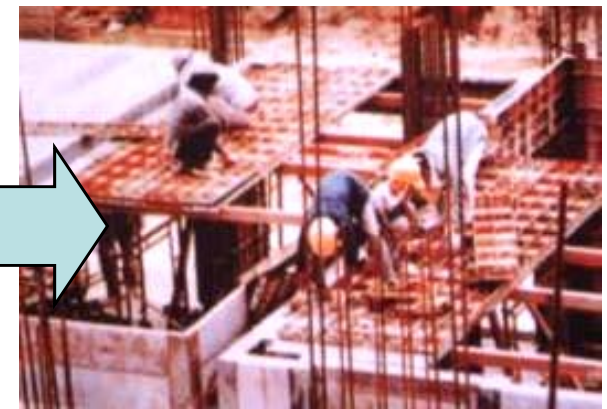
Timber Form to Metal Form
