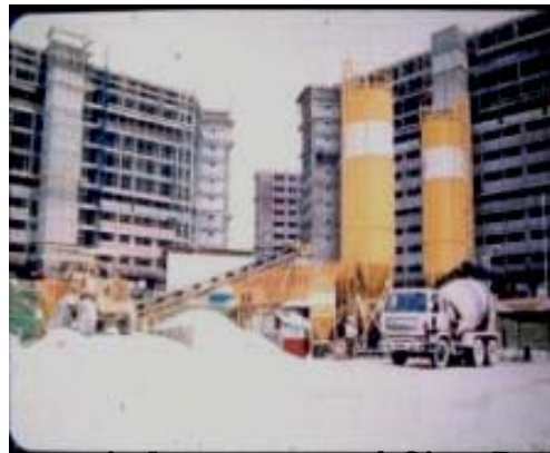
Semi-Automated Site Batching
